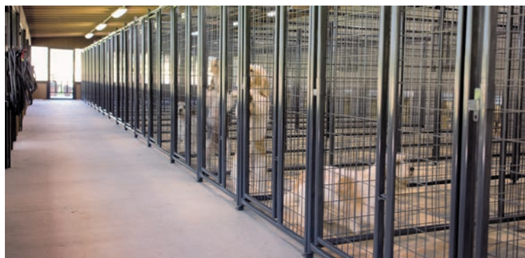
The outside runs of this dog kennel are enclosed by protective screening to help reduce the infiltration of insects, such as kissing bugs.
